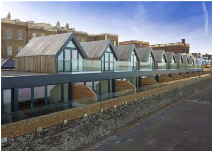
Beachside House, timber rain screen and Gabions filled with pebbles ABIR Architects
